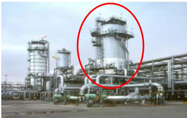
Figure D2: Saudi Aramco Econamine (DGA) Plant in Uthamaniyah, Saudi Arabia – The absorber (center-right) has a 40-foot diameter
