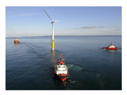
The world's first large-scale floating wind turbine is located approximately 12 km south east of Karmøy in Norway at a water depth of about 220 meters.
