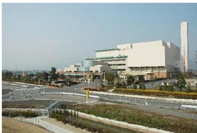
Fig.2 Waste Power Plant in Takagise Town (Source: Toshiba web site 2 )
