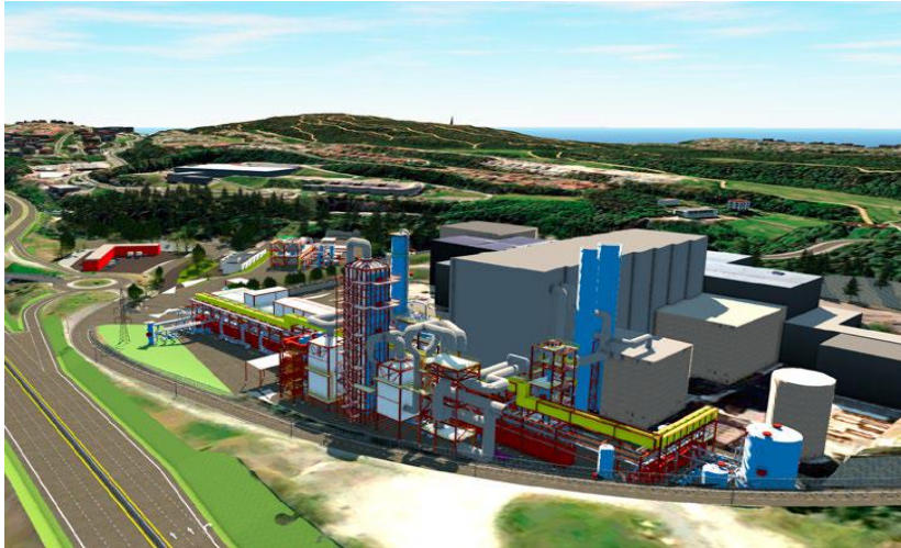
Fortum Oslo Varme's existing plant (shown in grey) and the planned capture facility (in other colours). Source: Fortum Oslo Varme AS
