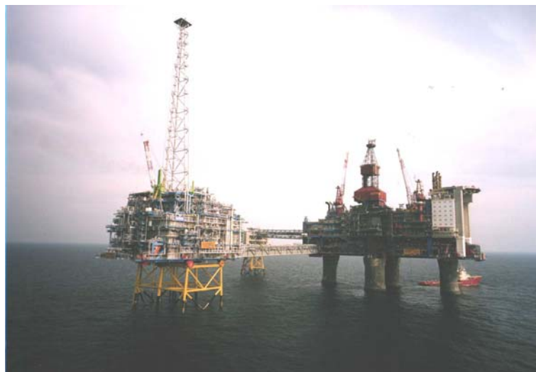
Figure 45. The Sleipner Platforms. The platform on the left is the Sleipner T gas-processing platform, where the CO 2 from the Sleipner west field is separated from the methane. The concrete-legged platform on the right is the main Sleipner A production platform from which the CO 2 is injected underground via a 3 km long deviated well, see Figure 46. (Photo Statoil).
