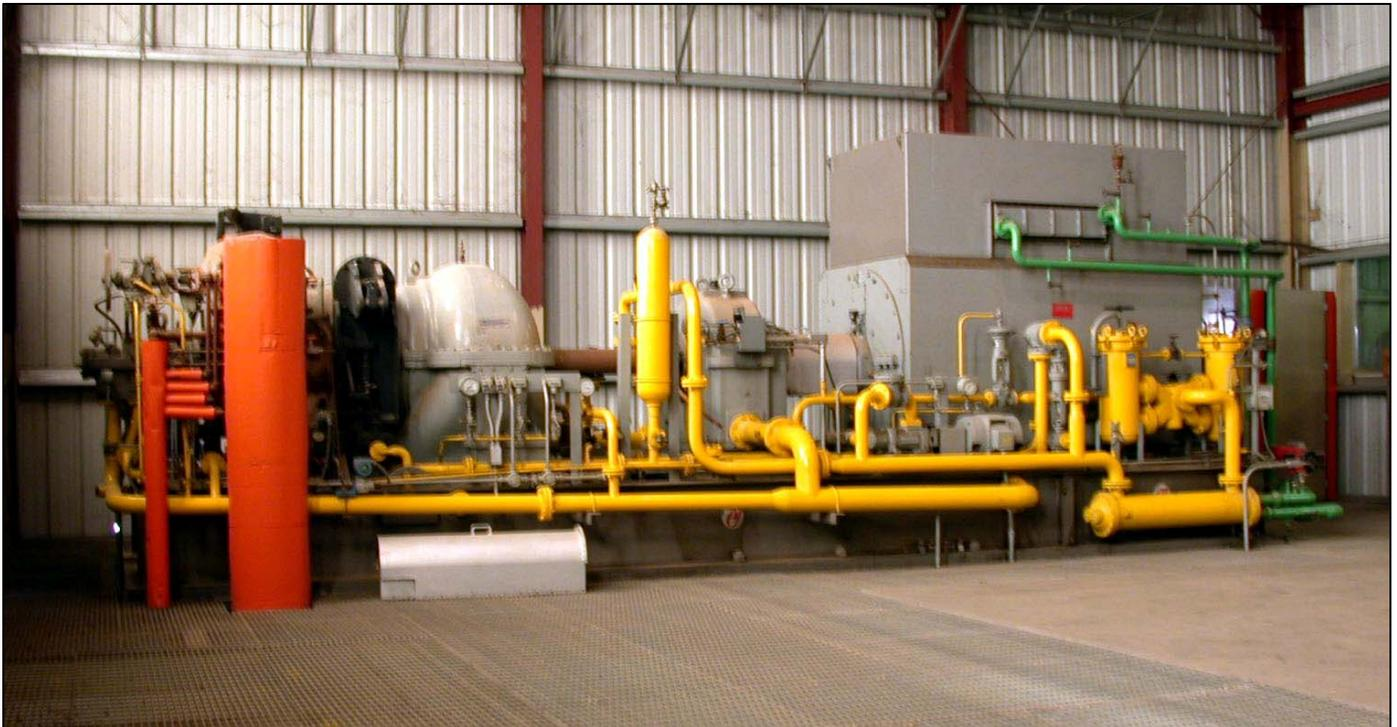
**5.5 MW Steam Turbine (operating on a steam/CO<sub>2</sub> drive gas) and Generator**
