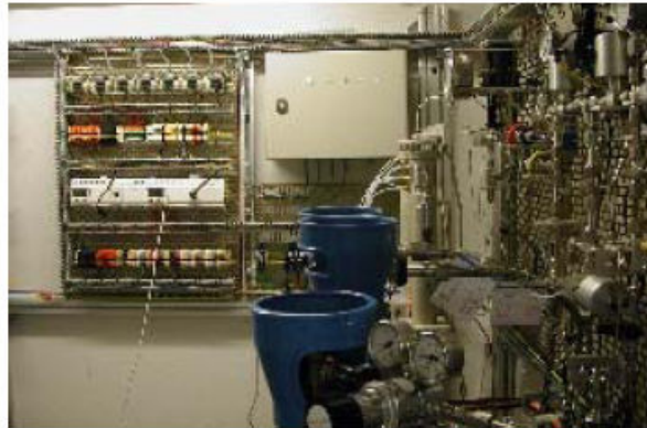
Controls and Electronics
