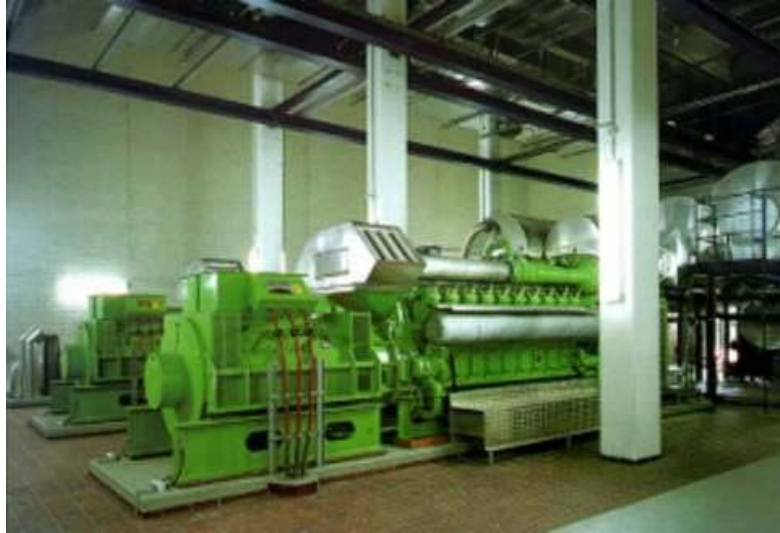
Figure 2-4. Reciprocating engine > 1 MW e (Jenbacher J620)
