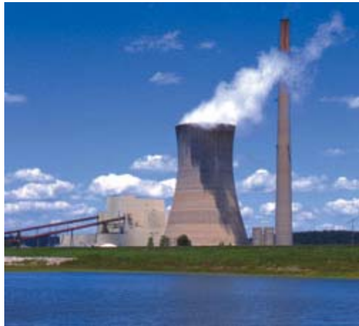
Mountaineer Plant - New Haven, WV
