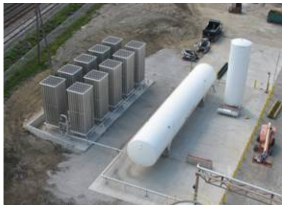
11,000 gal and 52,000 gal LOX tanks installation
