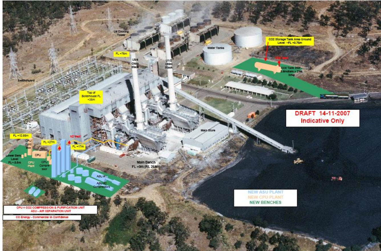
CALLIDE OXYFUEL PROJECT VISUAL AMENITY - AERIAL VIEW FROM NORTH EAST OF CALLIDE A
