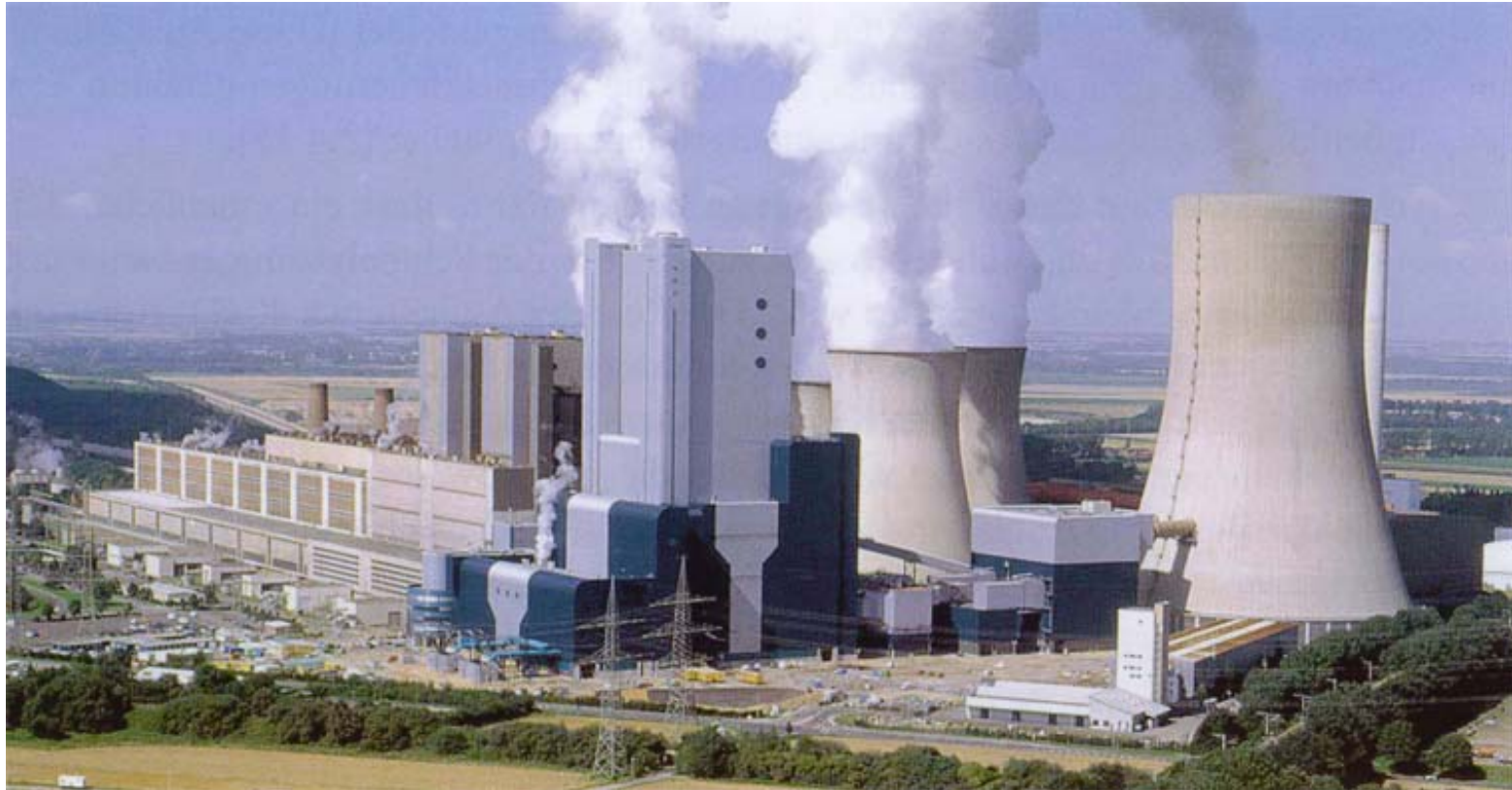
Block K, 1012\text{MW}_{el} , net efficiency over 43 %, lignite coal, RWE Power, Niederaussem, Germany
