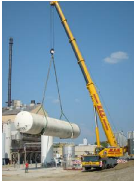
11,000 gal and 52,000 gal LOX tanks installation
