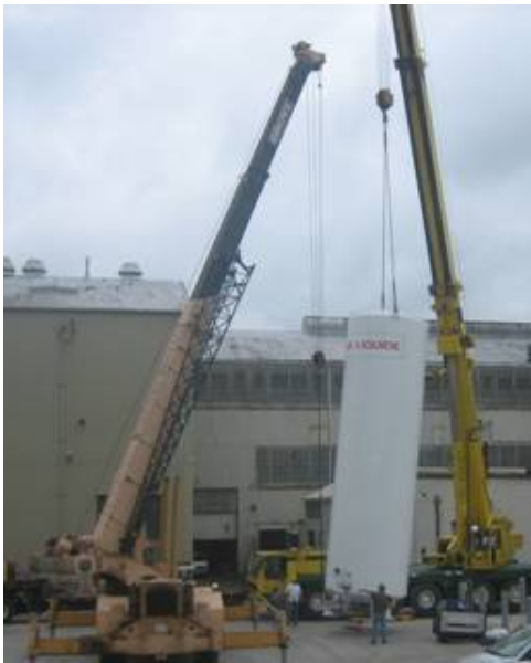
11,000 gal and 52,000 gal LOX tanks installation
