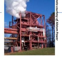
$15\,MW_{th}$ oxy-coal combustion unit
