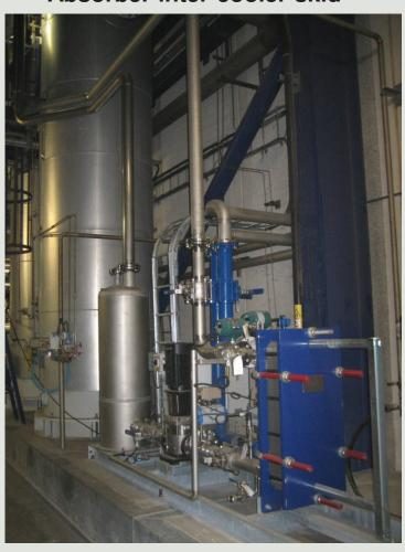
Flash vessel for vapour recompression
