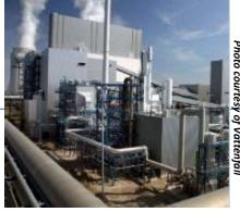
50+MW<sub>e</sub> oxy-fuel **Demonstration**
