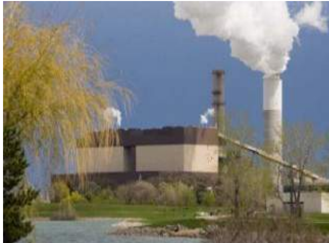
Pleasant Prairie Power Plant ("P4")
