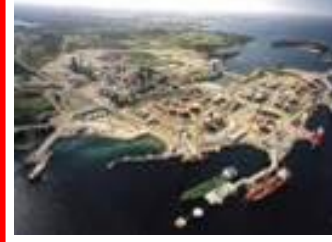
TCM Mongstad Norway - 40 MWth Chilled Ammonia - Gas
