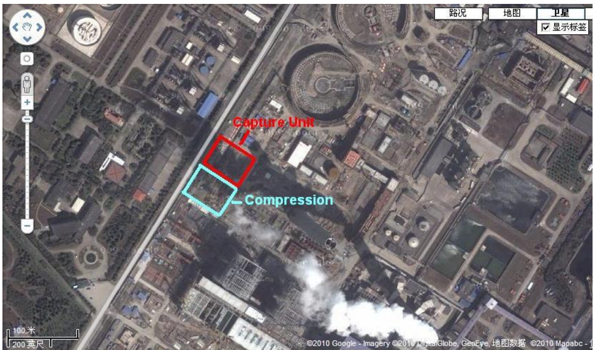
Figure 6.10 Shanghai Shidongkou retrofit unit (this figure shows the unit while it is still under construction)
