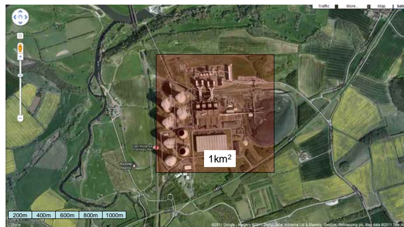
Ratcliffe-on-Soar Power Station UK. Main plant area ~ 1km 2 , capacity 2GW
