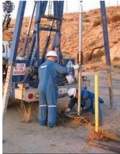
*This flux tower being installed at a geologic storage site measures the concentration of gases in the atmosphere. Such devices can detect increases in CO<sub>2</sub> Image source CO2CRC*
