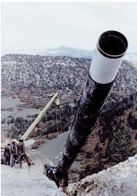
Figure 17 - Placement of Cortez CO 2 pipeline section (Willbros, 2013)
