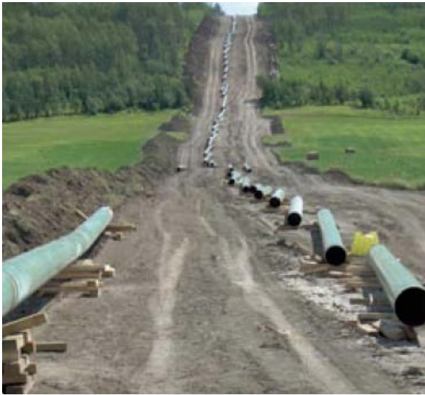
Figure 16 - Stringing and welding of pipeline (Shell, 2010)
