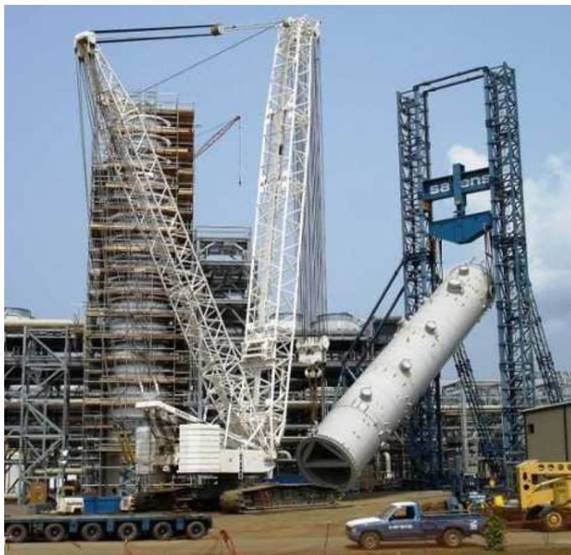
Figure 7-1: Reactor installation with gantry crane (example)
