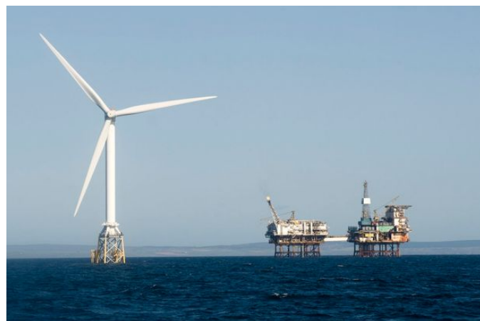
Figure 9-6: Beatrice AD and AP Platforms with one of the 5MWe turbines
