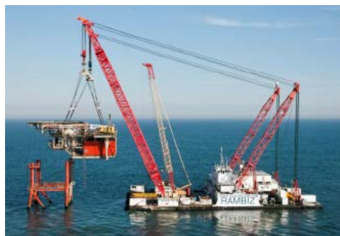
Figure 5-5: Removal of the Camelot A Topsides
