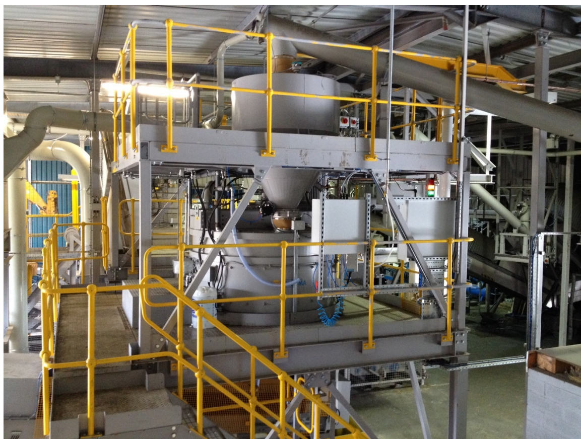
Figure 4.5 First stage vessel at the Carbon8 Brandon facility
