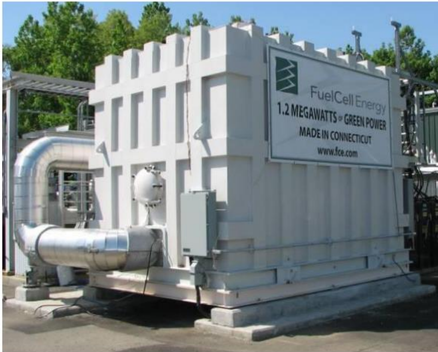
Figure 38: Typical MW-scale FC Module by FCE (Ghezel-Ayagh, 2017)
