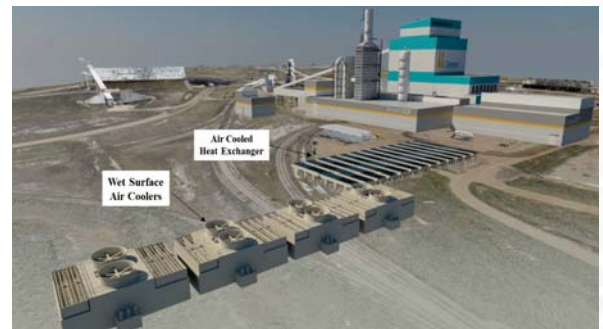
Figure 10. Proposed new hybrid heat rejection system
