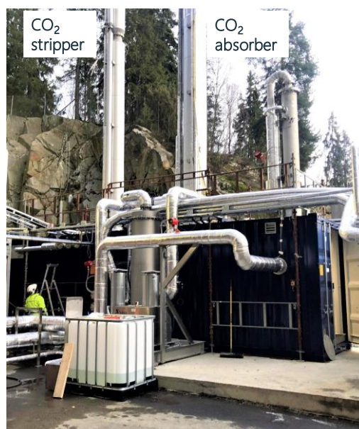
Figure 47: Fortum Oslo Pilot Plant for CO 2 Capture from WtE. Source: adapted from Bjerkas, 2019.
