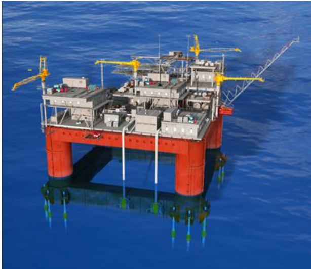
Figure 10-10 Tension Leg Platform (TLP) 375
