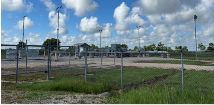
ExxonMobil's Green Pipeline at the Beaumont ump station
